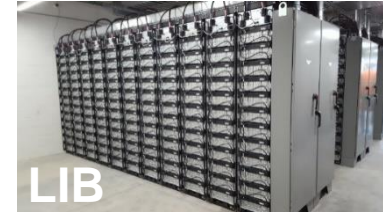
AltaGas 80MWh Li-Ion battery installation: http://www.marketwired.com/press-release/altagas-celebrates-opening-of-north-americas-largest-battery-storage-facility-tsx-ala-2191585.htm
